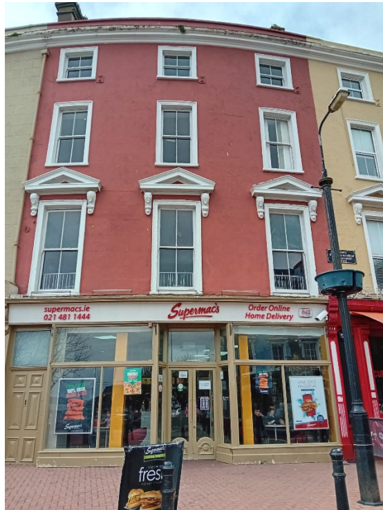
2 Casement Square – Jack and Shiela
